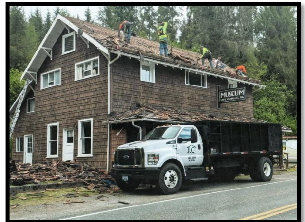
Lupo Crew: Work in Progress
